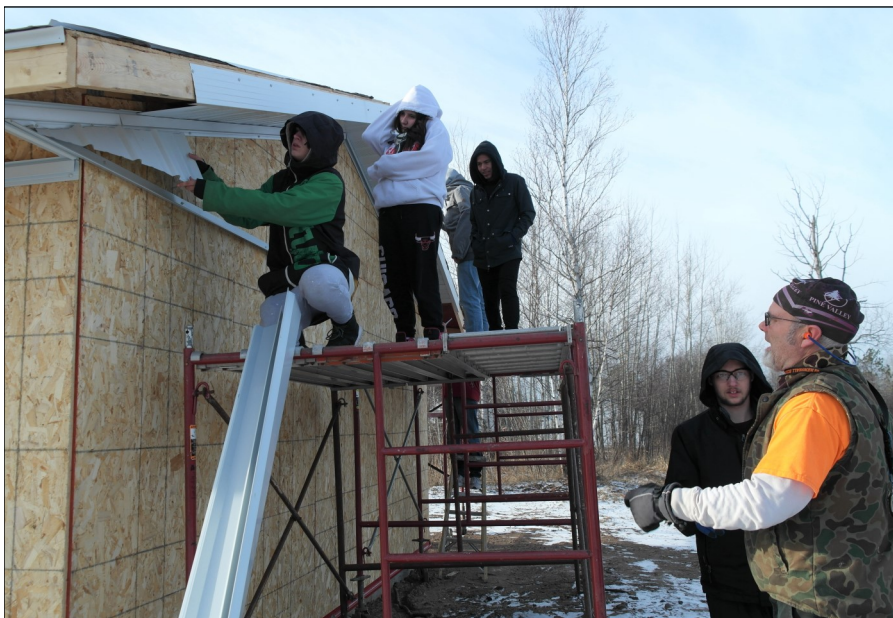
Construction Class Teacher Chris Gustafson advised students as they worked on building the new recycling center in Mahtowa.
