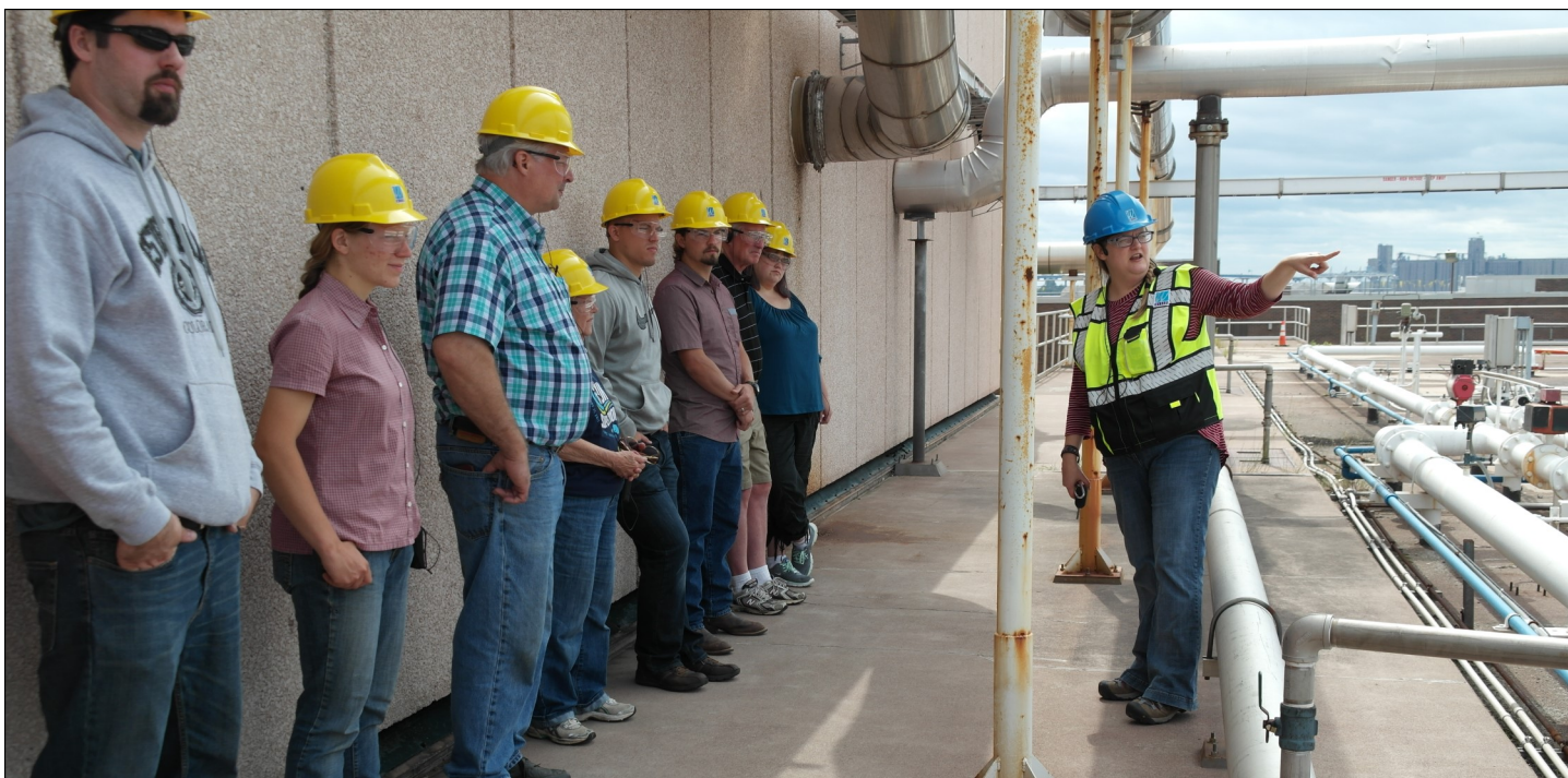
Lerohl informs SWARA Committee members on the steps of the water treatment process.
