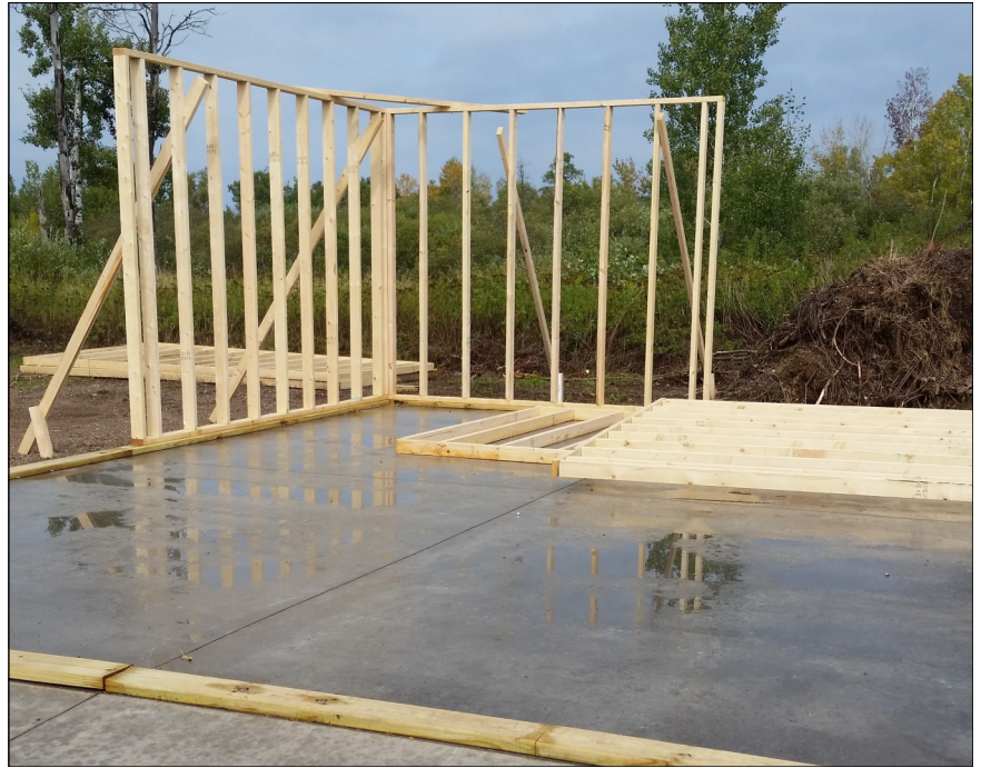
Concrete has been poured at the site, and the walls are being built off site.
